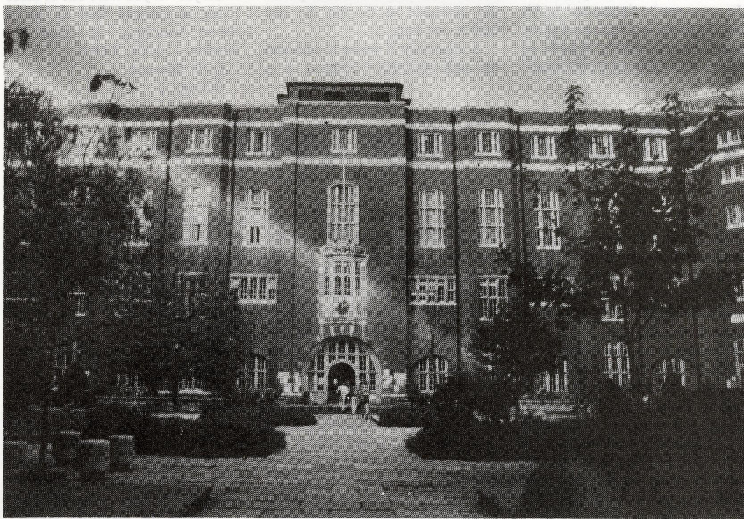
The Union Building, recently refurbished at a cost of £60,000
