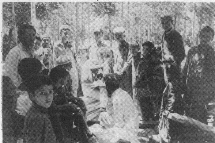
Henry interviewing on the building site
