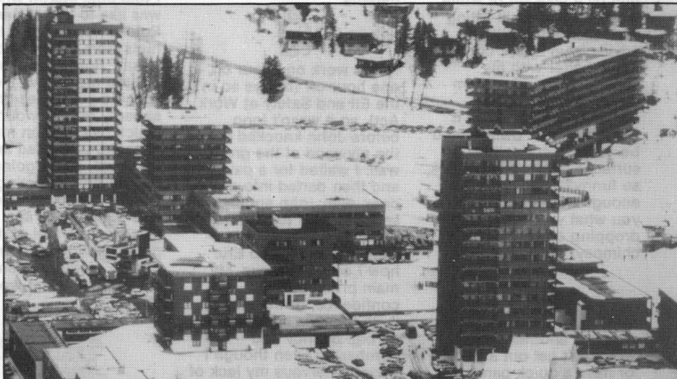
Tower block apartments at La Plagne, France
