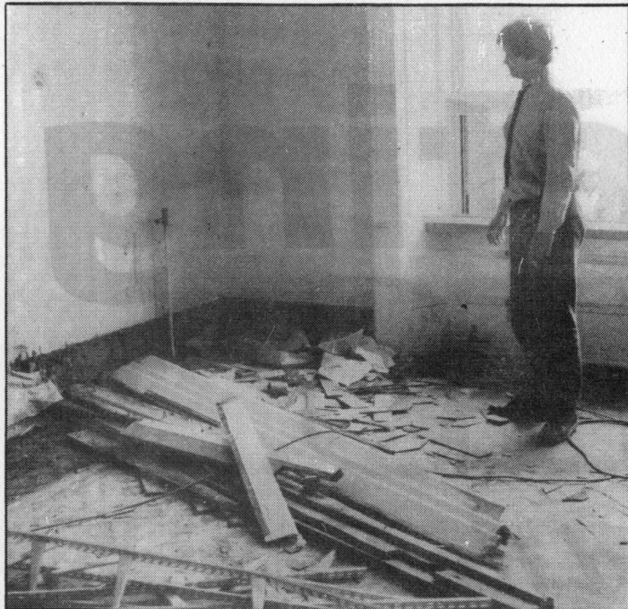
Michael Arthur surveys the damage.
