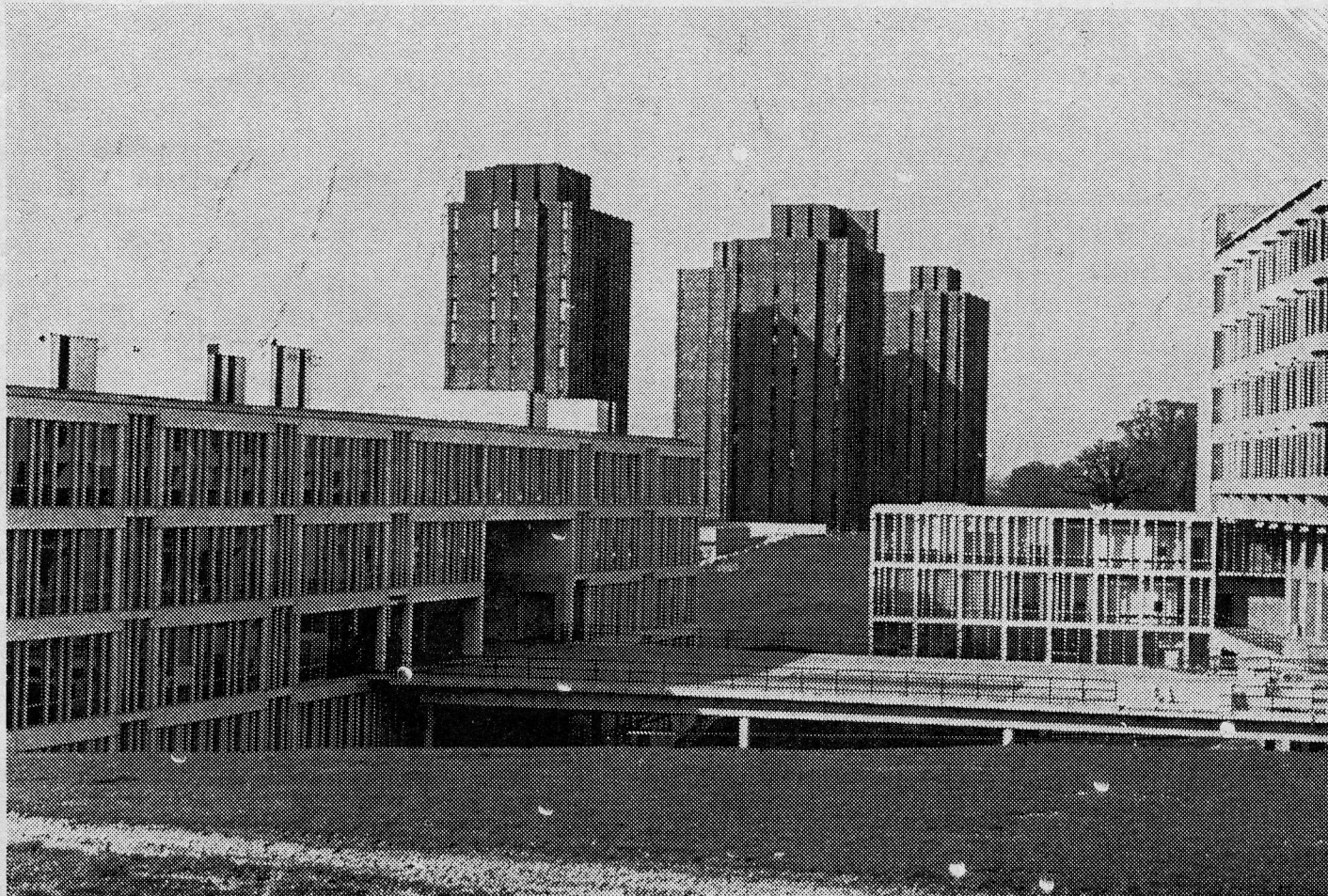
The towers, seen looking north
