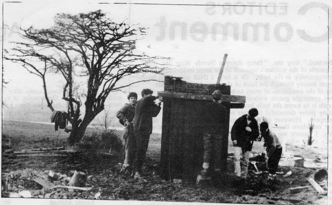
Building the "rabble tower" in record time.
