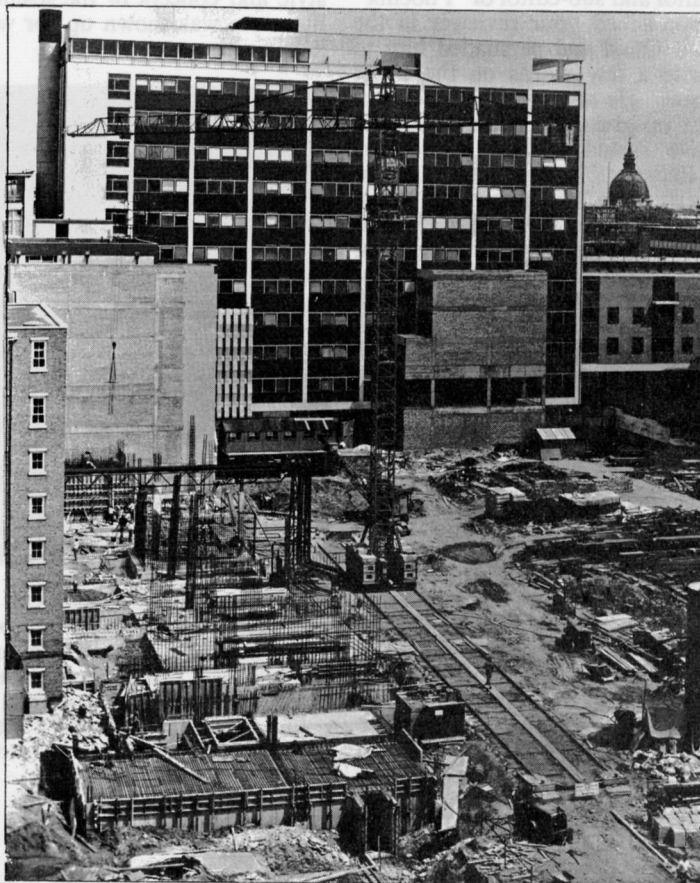
The Aero and Chem. Eng. Extensions under construction. Summer 1964.
