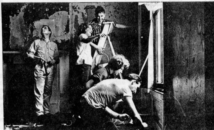
Renovation in Progress in Notting Hill
