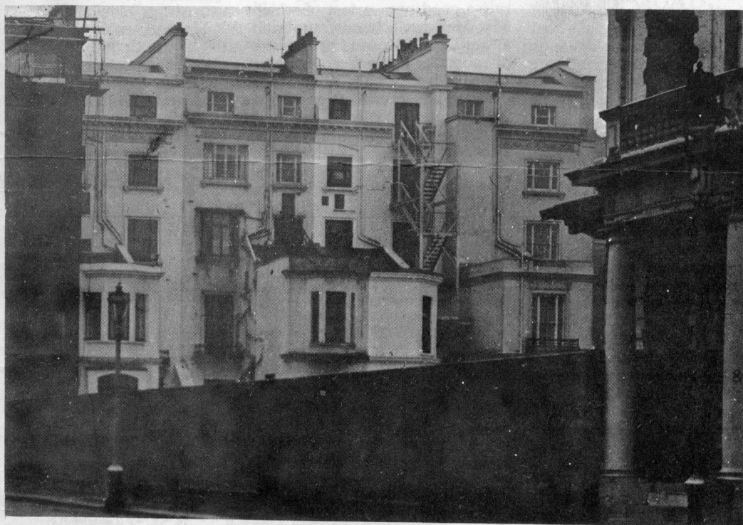
The Site of the Sports Centre ; North Side, Princes Gardens.
