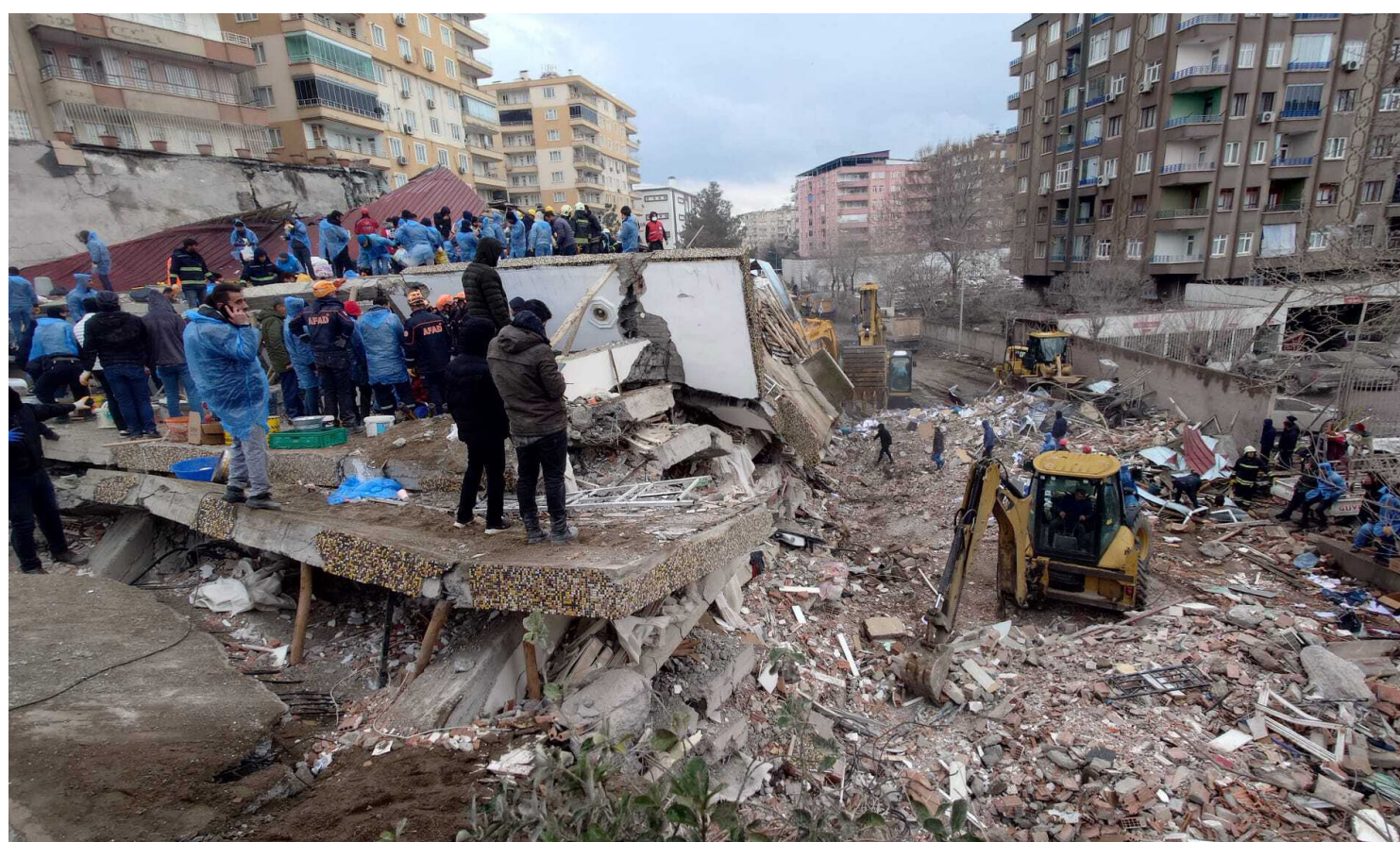
Cleanup of the wreckage of a collapsed building in Diyarbakir, Turkey, following the 7.8 magnitude earthquake which had its epicenter in Gaziantep. Stemoc / Wikimedia Commons User (Licence: PDM 1.0)
