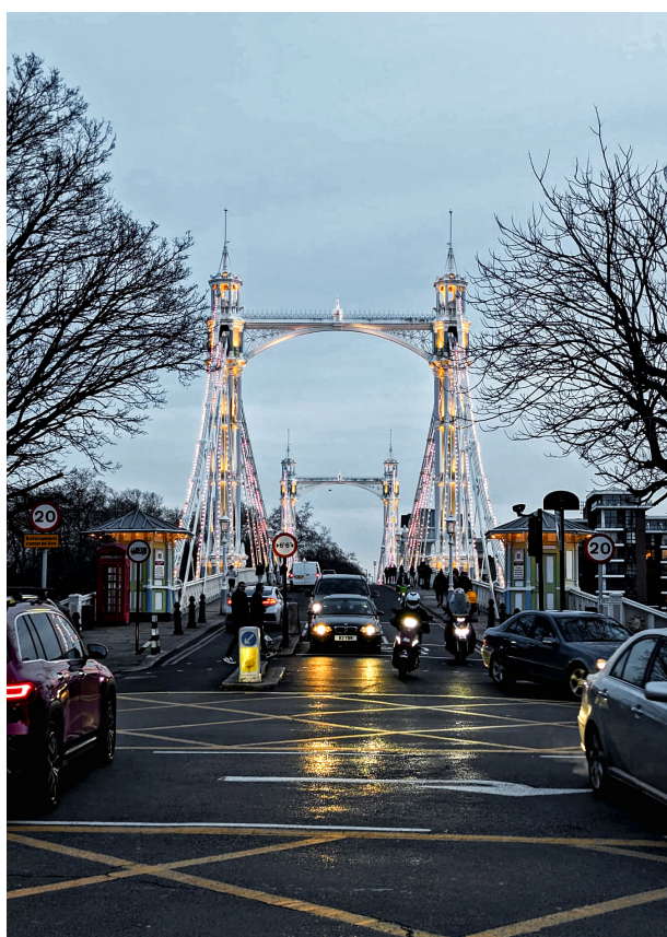
Looking down the Albert Bridge Zanna Buckland
