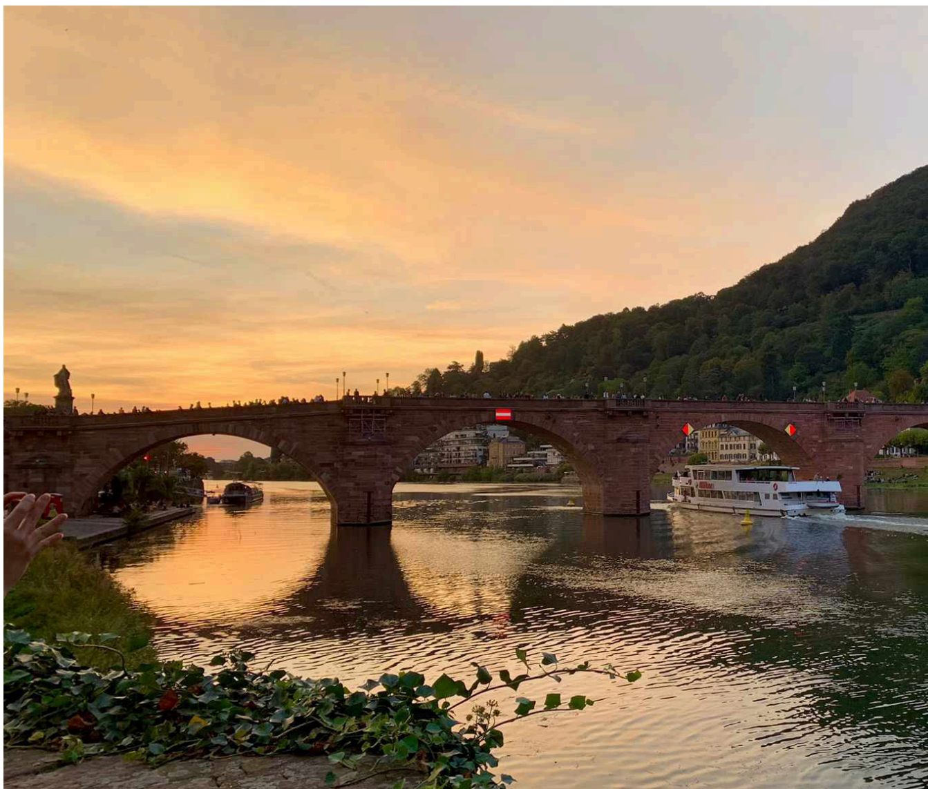
The Old Bridge Clara Maton
