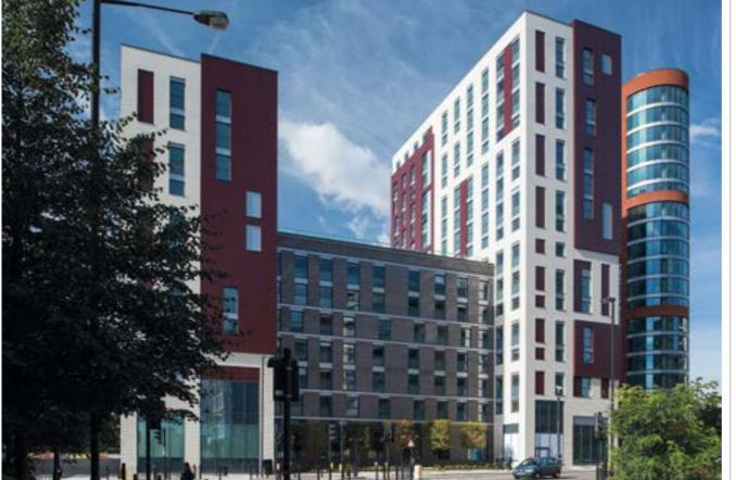
Woodward Buildings continues to have cladding that has failed fire safety tests // Imperial
