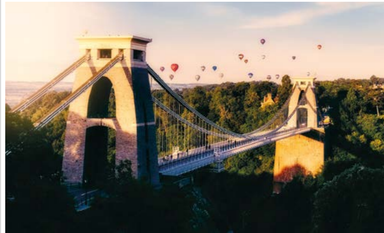
Clifton Suspension Bridge is a must for your travel bucket list // Pixabay
