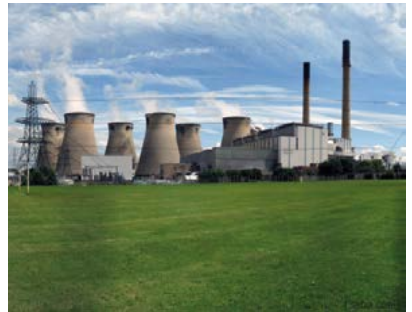
Ferrybridge Powerstation, UK, where the experiments took place.
