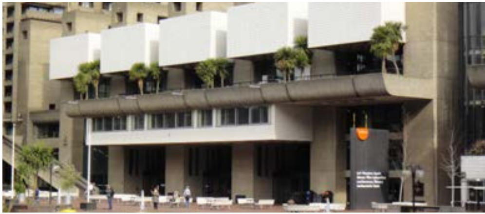
The brutalist facade of the Barbican Centre, London's largest arts centre Photo: Creative Commons
