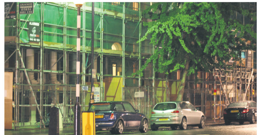
Albert Hall Mansions laden with scaffolding, where the mugging took place
