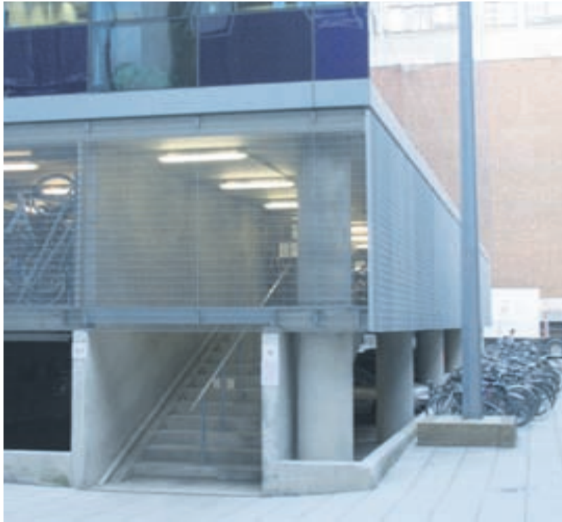
Turnstiles will be installed in the entrance to the Faculty Building bicycle store over the Easter break
