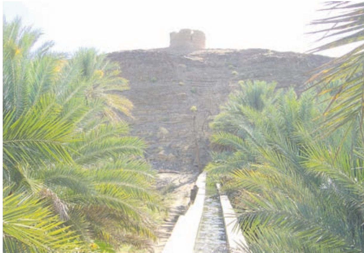
Part of a Falaj system in Oman – an ancient system that taps in to shallow groundwater and feeds it to the surface. Some aflaj are more than 1500 years old; as a whole they've been deemed a World Heritage Site
