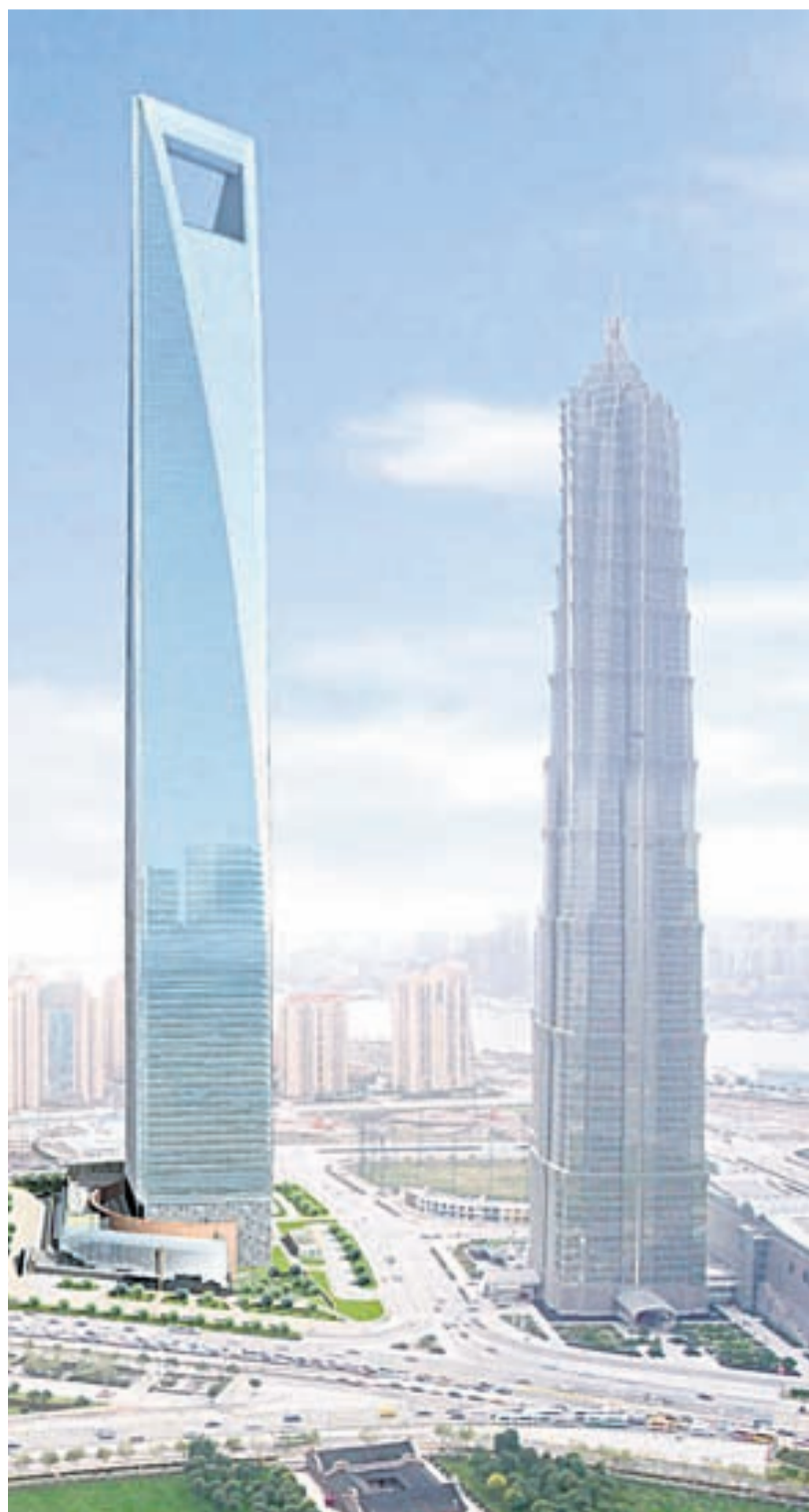
Shanghai International Finance Center (adjacent to the Jin Mao tower)
