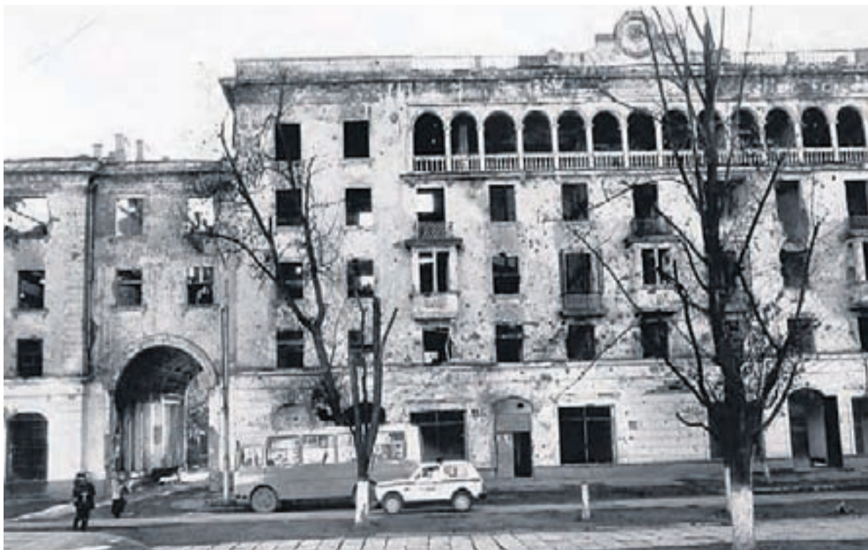
A shelled out building in Grozny, capital of the troubled Russian state of Chechnya
