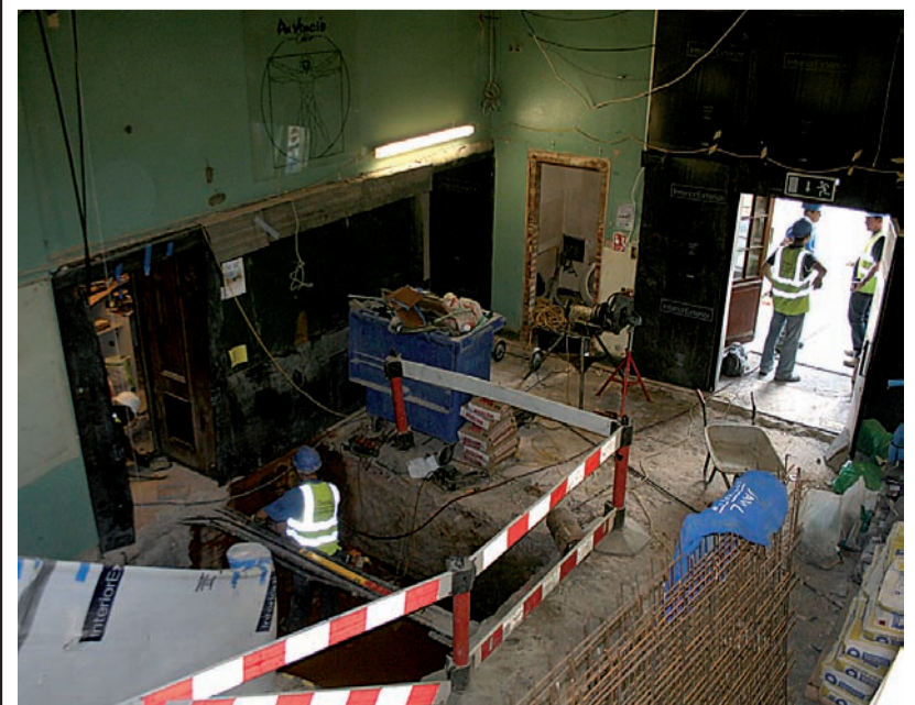
The core of the Union building, showing the lift excavation
