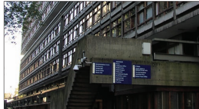
Southside: set for demolition this summer
