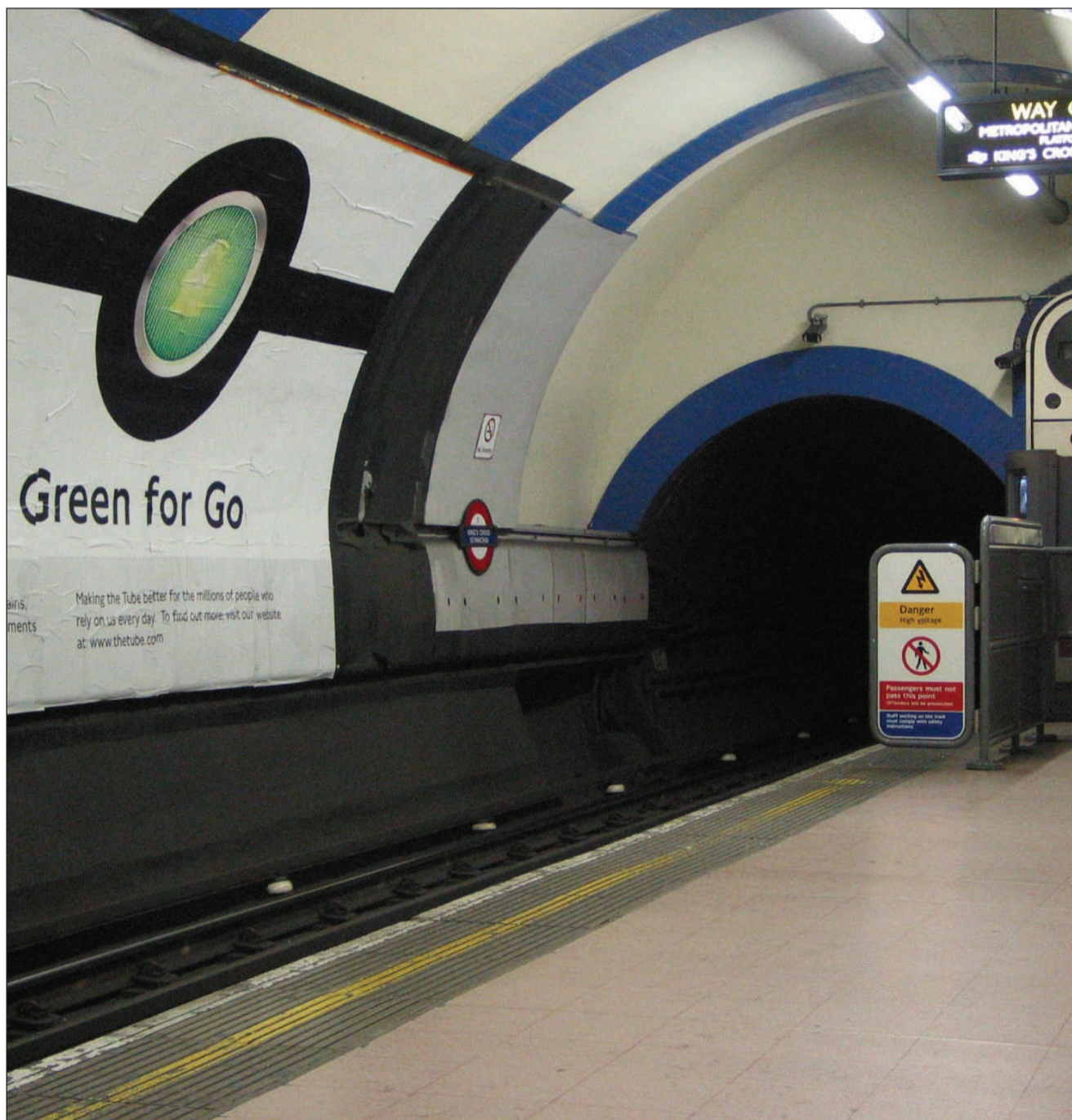
The beginning of a long mission: Transport for London prepares itself for a 30-year transformation of its infrastructure
