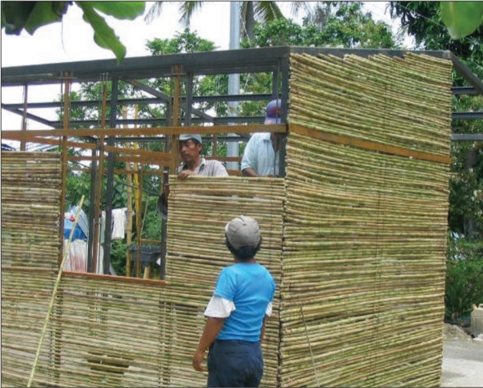
9. Fix the barras to the structure
