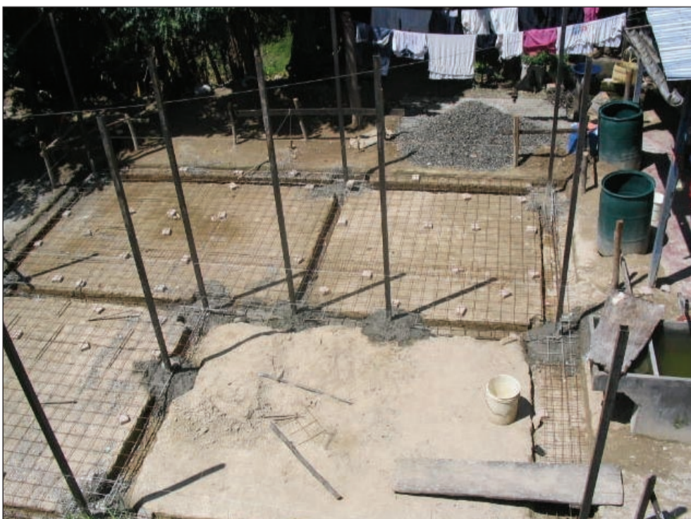
5. Dig trenches and column footings. Concrete the house's frame into place
