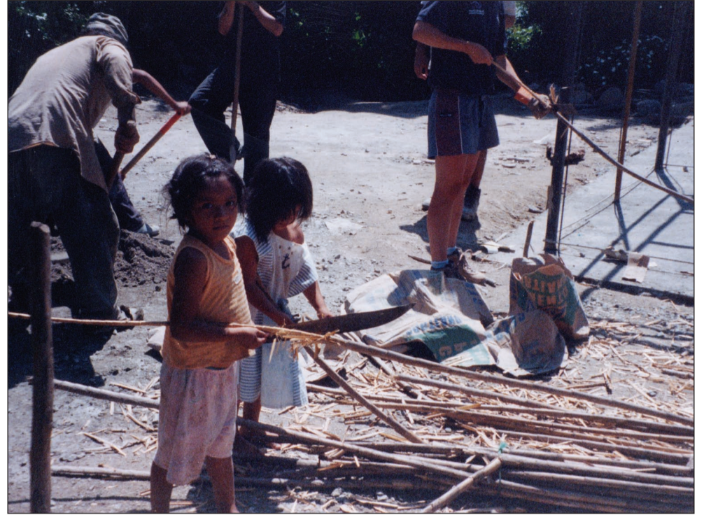
8. Prepare 'barras de castillas' to line the walls with. Using small children if needs be
