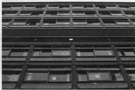
Southside: looking up?
