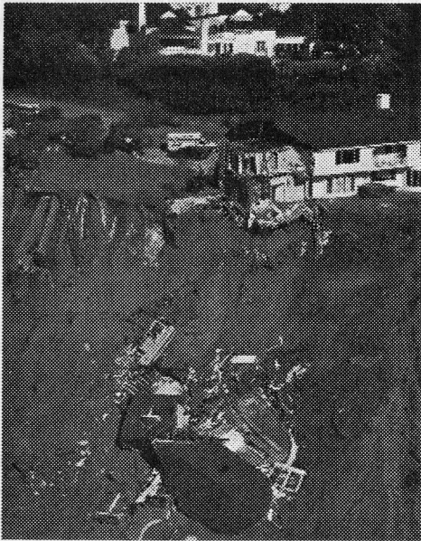
House Destroyed in 1994 Northridge, California Earthquake.
