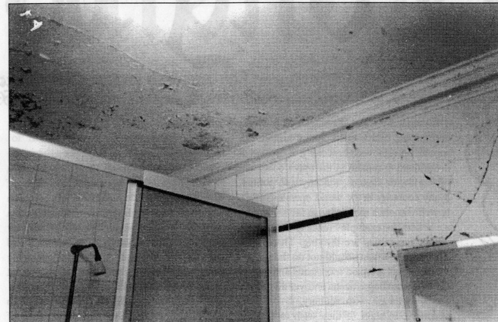
The inviting interior of Fisher Hall's showers. Students share their daily ablutions with flakes of paint, mould and mushrooms.
