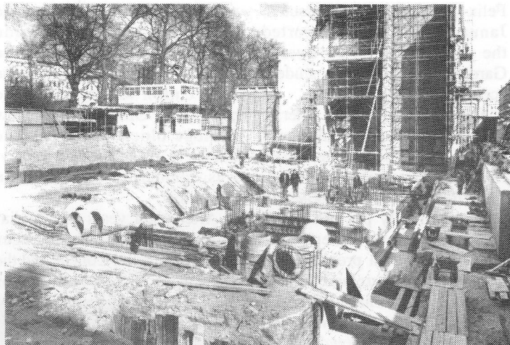
The Sports Centre under construction in 1967
